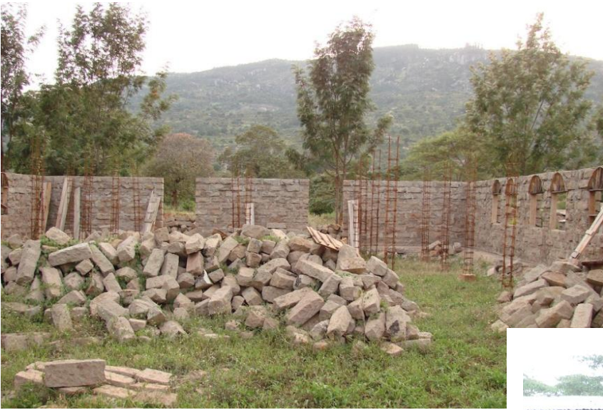
Hand cut stones used for the wall
