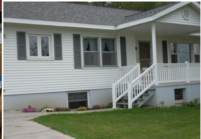
David completed our new front porch
